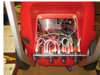
Control Panel - Open
