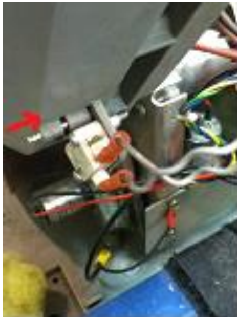
Trap Door pin being pushed to secure trap door in place.
